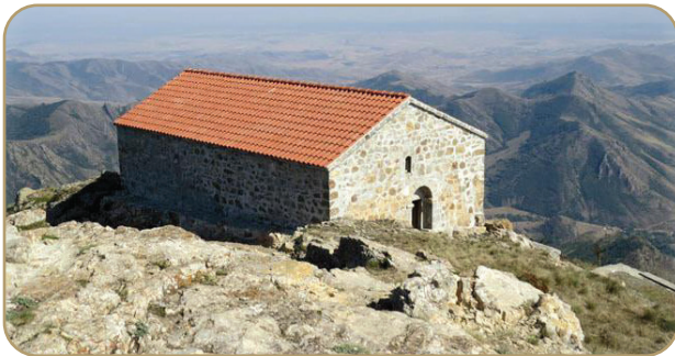
After the illegal reconstruction, the Armenians presented this monument as an Armenian church.
