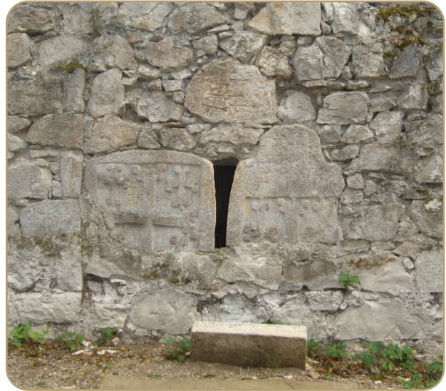
A number of ancient cross-stones were used to build the walls of the Urekvank Monastery.
