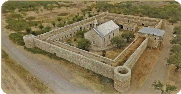
The Amaras monastery complex is surrounded by rectangular fortress walls with round towers at its four corners.
