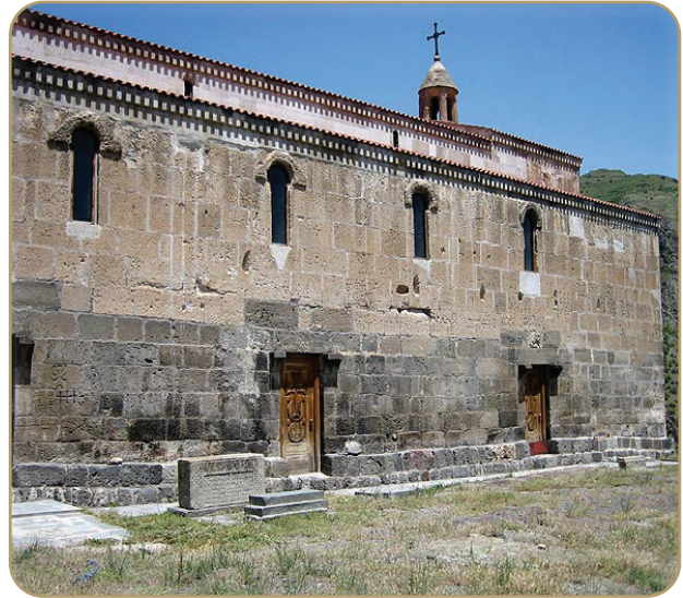
For the purpose of illuminating the temple's interior, the walls have long, narrow windows.
