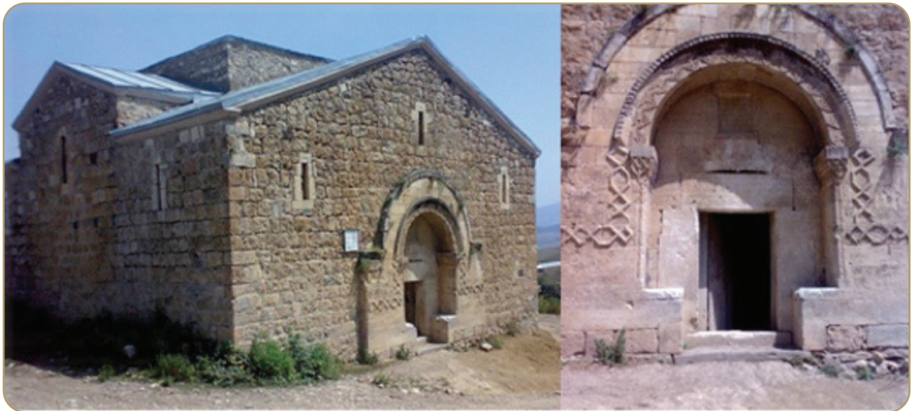
Albanian church (14th century), Kharkhar village. During the occupation, unlawful repairs were made to the monument, causing the church to lose its historical appearance
