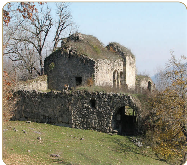
The Great Arran monastery complex consists of two churches surrounded by fortress walls, two narthexes and auxiliary buildings
