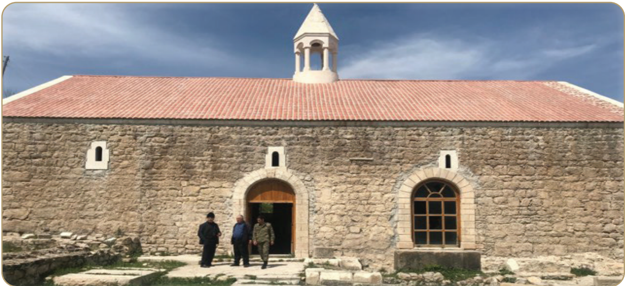
St. John's Church, 2021. The church's original look was altered when it was subjected to illegal restoration work by Armenians during the occupation, and a great number of gravestones taken from elsewhere were erected around it.
